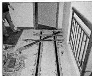
CFRP Strengthening
