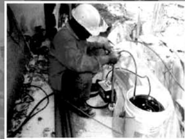
Geotechnical Instrumentation Installation & Monitoring
