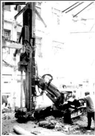
Bored Micropile Installation at Conservation House
