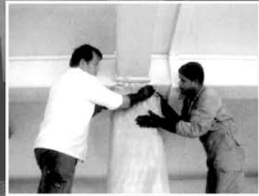
Column Strengthening by FRP System
