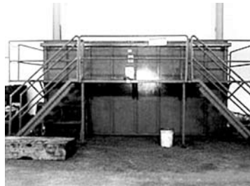
Varnish Dipping Tank c/w Safety Railing
