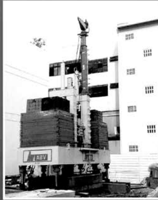
Jack In RC Pile in Residential Area
