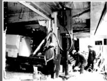
Driven Patented Steel Micropile within Low Headroom Building
