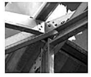
Pre-tabricated Truss for Easy Installation
