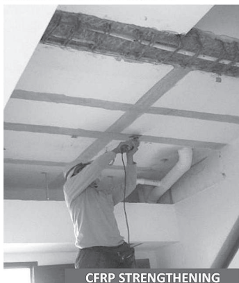
CFRP STRENGTHENING
